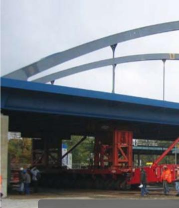
Case study: Jack-up and installation of a bridge, Germany
