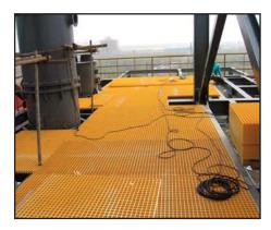
These pictures show examples of fibreglass grating installations. Fibreglass grating has the added advantage of quick and easy installation on site.
