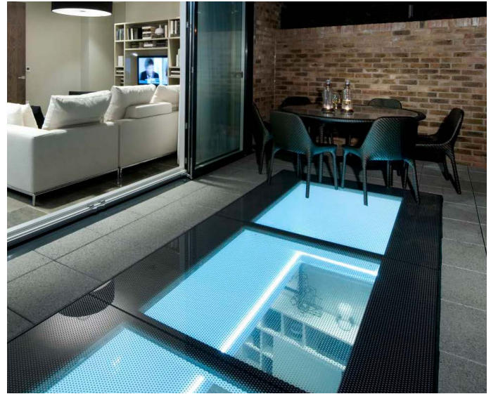
Example of typical anti slip frit pattern applied to walk on glass.
