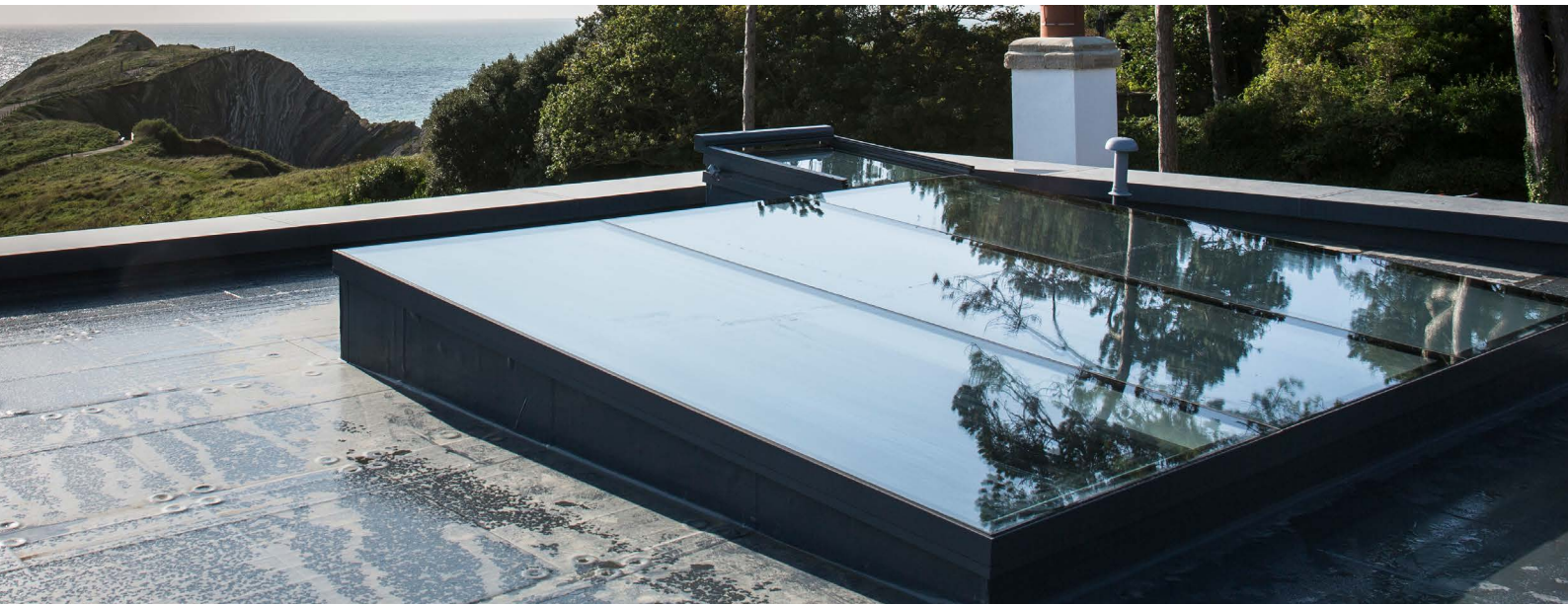
Partially shaded rooflights can be susceptible to thermal heat stress unless the correct glass specification is used.
