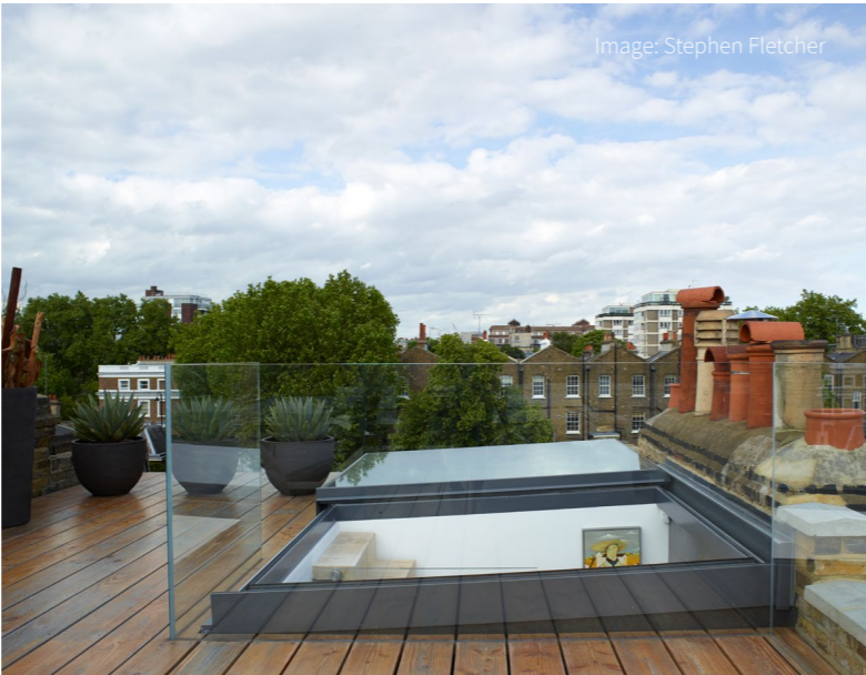
Examples of safety barriers being installed for edge protection and to prevent building occupants falling into void created by access rooflights.
