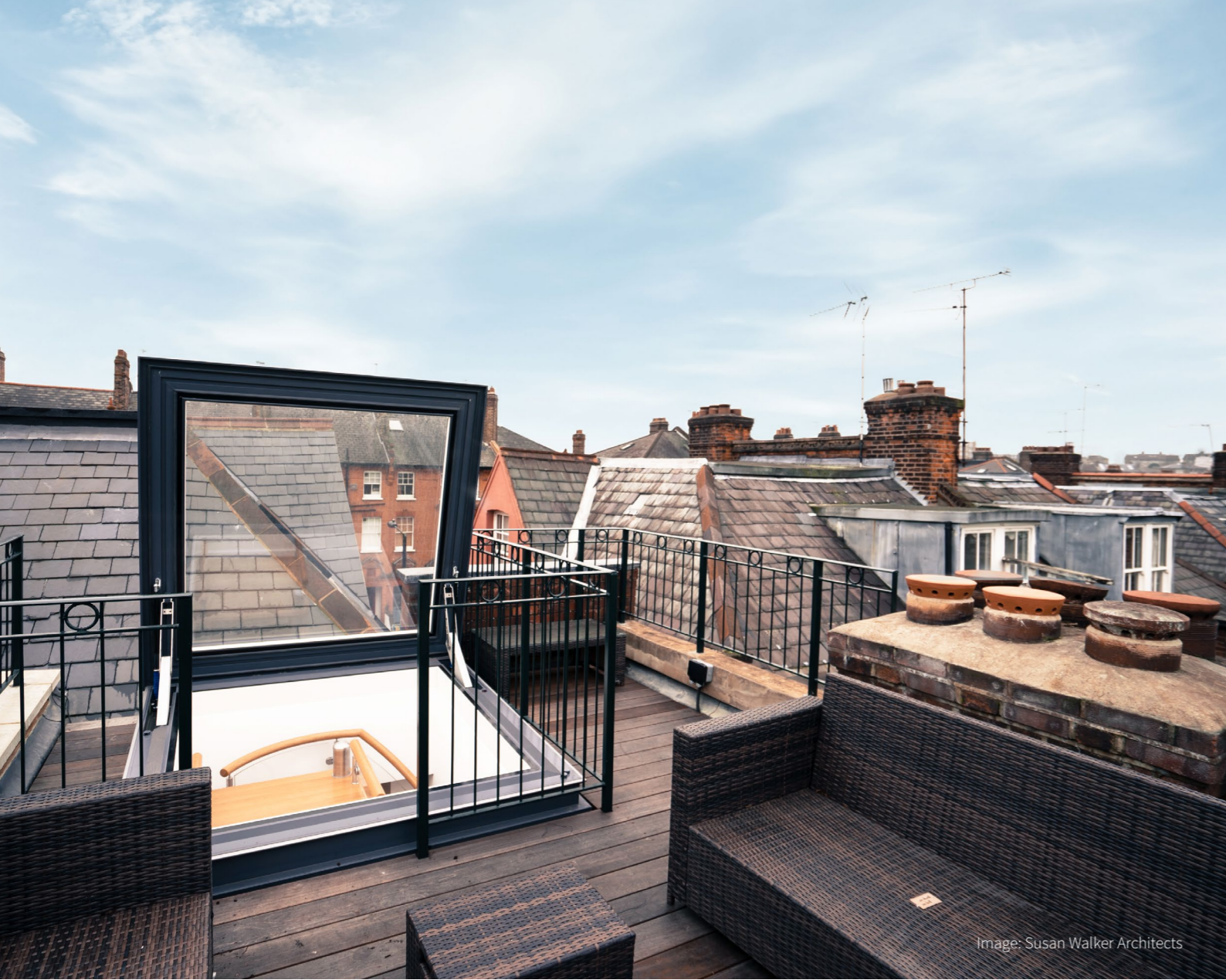
Examples of safety barriers being installed for edge protection and to prevent building occupants falling into void created by access rooflights.
