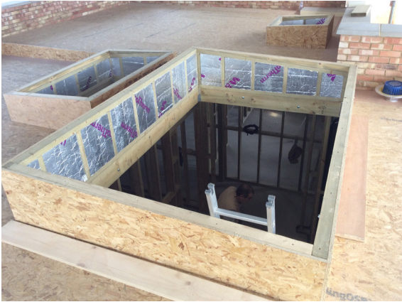
Structural rooflight upstand for flat roof.
